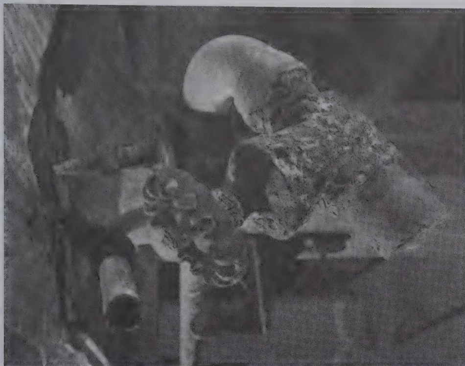
Figure 5.3 Tap were rendered useless by heavy mineralisation
